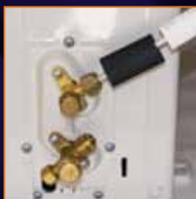
5. Installation of standardized flare nut (tightening torque acc. to A/C unit manual)
