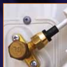
5. Installation of TALOS DUAL flare nut (tightening torque acc. to A/C unit manual)
